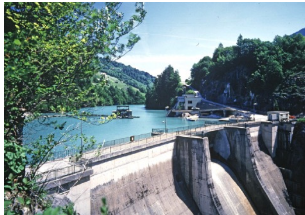
Existing hydroelectric dam "Lower Lutz", Raggal, built 1956, volare 2004
